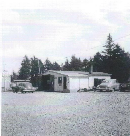
Eisenhauer White Rose Service Station (Located across from present day Glen Arbour)- 1956
