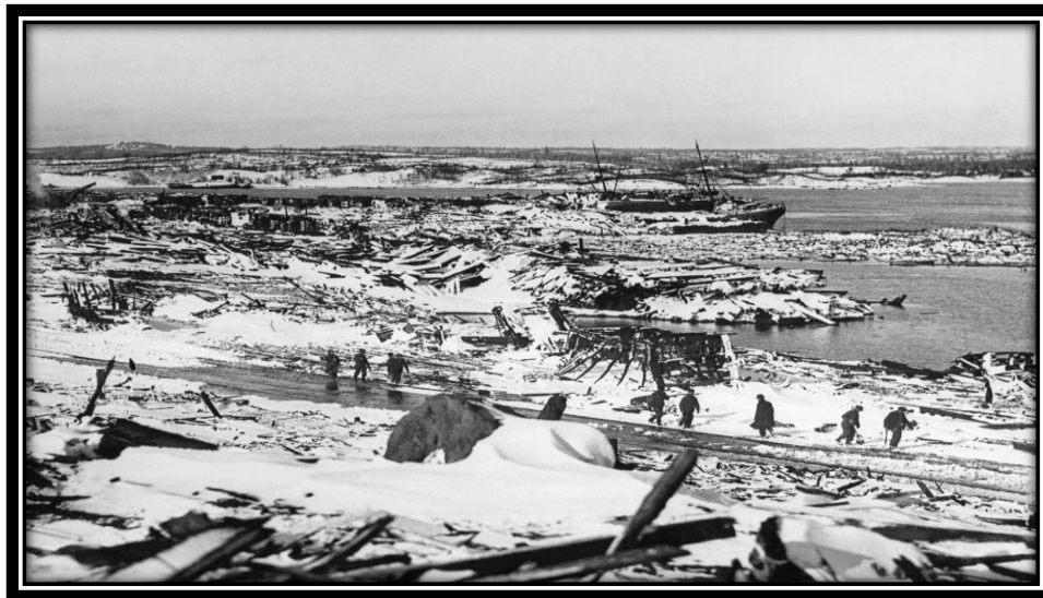
A couple of views of the destruction of the Halifax Explosion
