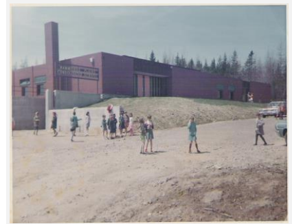
The new Hammonds Plains Consolidated School as seen soon after it opened – Spring 1968
